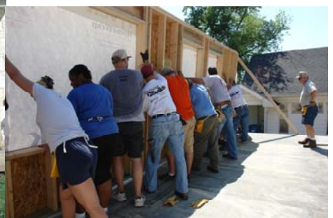
1116 E. Atchison Raising the Walls
