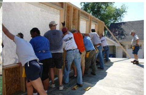
1116 E. Atchison Raising the Walls
