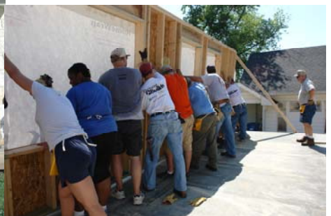
1116 E. Atchison Raising the Walls
